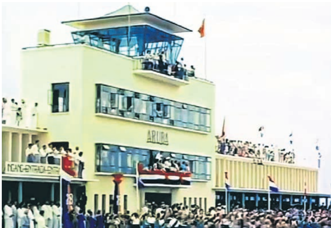
1955, third terminal building, arrival of Queen Juliana & Prince Bernhard
